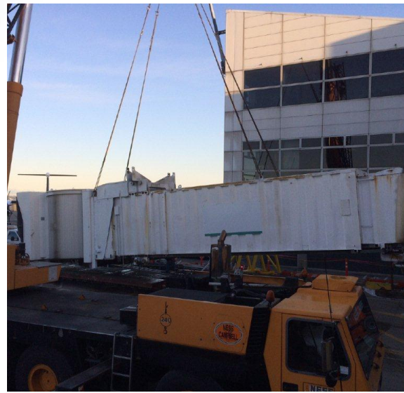
C12 Bridge Removal
