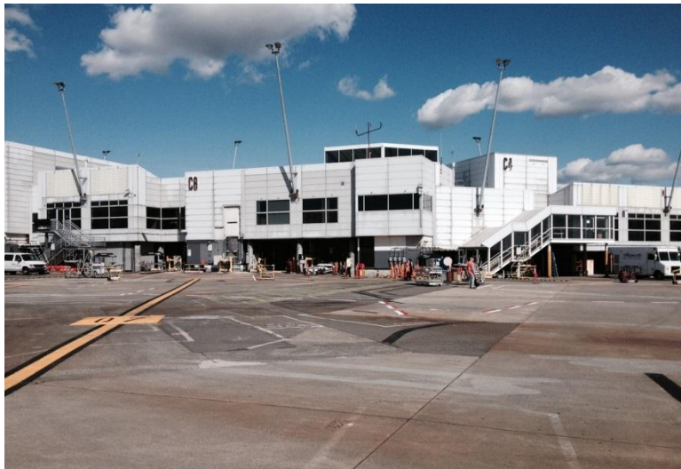
Where old C4 walkway Came Out
