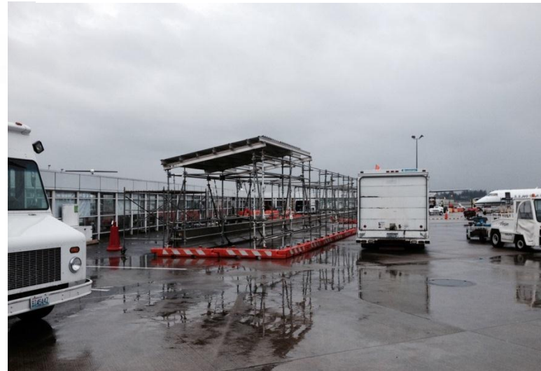
C2 Temporary Walkway
