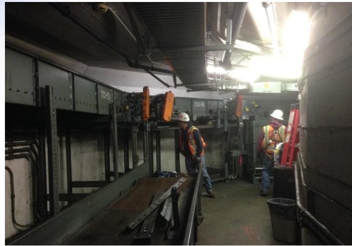
Power Turn in Progress
