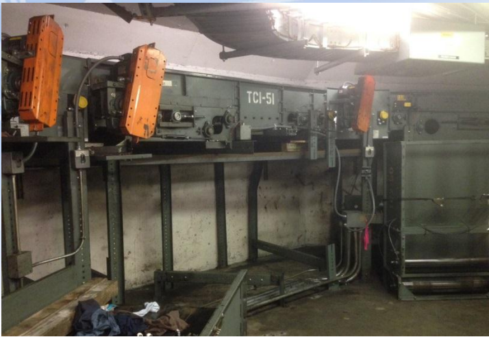
Power Turn Demolition
